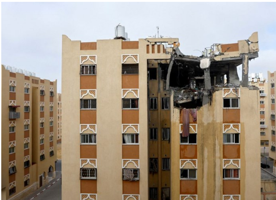
The destruction by the Israeli army of the building in which the commander of Islamic Jihad, Ali Ghali, was located
